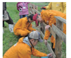
Constructing wooden fences in the Kiritappu Wetlands
