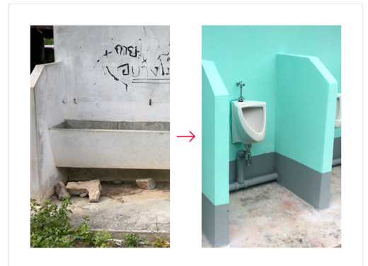
Upgrading of sanitary facilities
