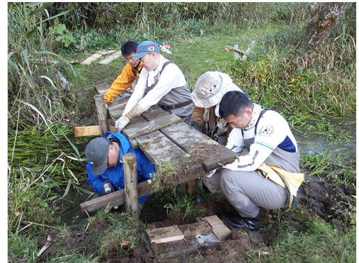
Constructing the wooden path
