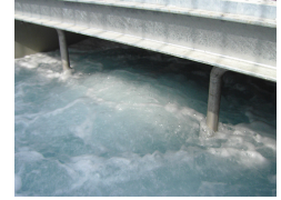
Hollow fiber membrane module unit (air diffusion)
