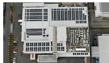
Kitakami Delica Plant solar panel facility
