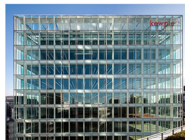
The double-skin glass facade of the Shibuya office.
